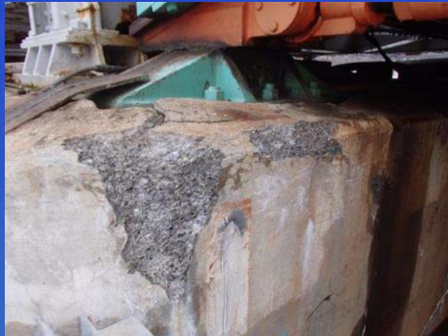
Spall in Pier 2 Cap
