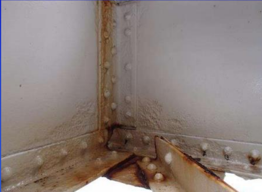
Pitting and Section Loss at Floorbeam – Truss Connections
