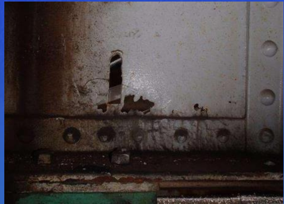
Perforations through Floorbeam Web in Span 4
