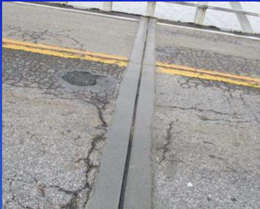
Top of Deck at Span 2 Contraction Joint
