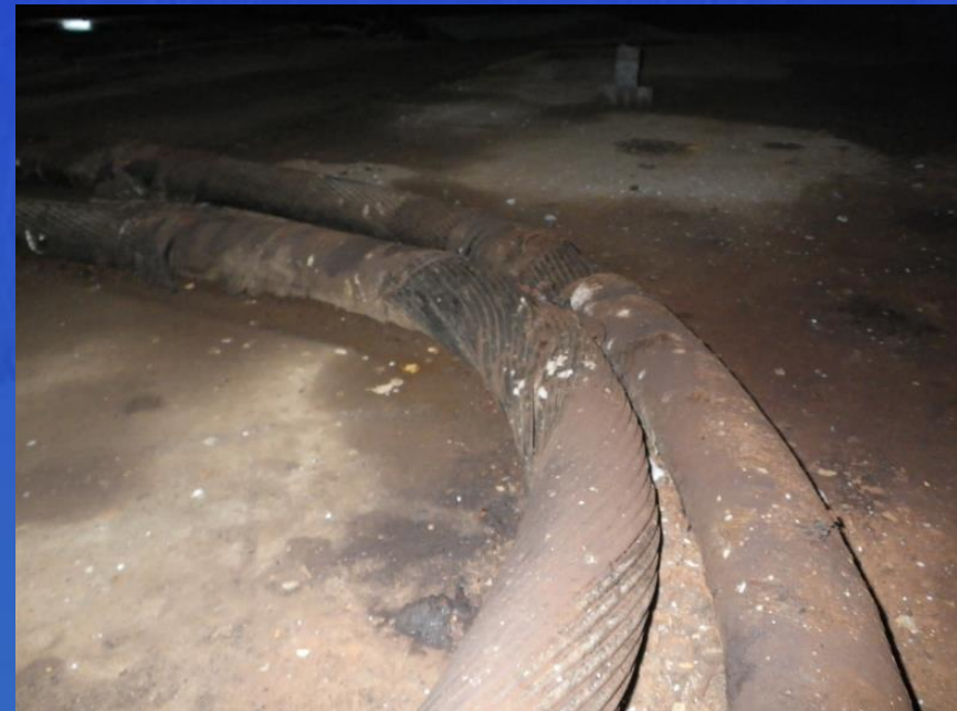
Submarine Cables Missing Protective Jacket
