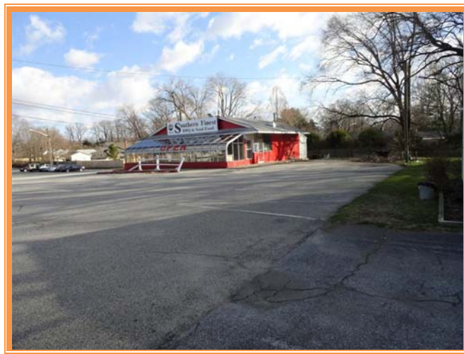
SIDE SOUTH VIEW
