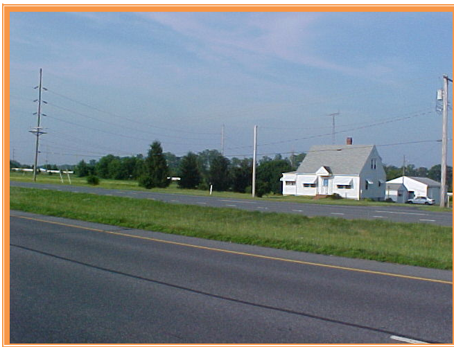
VIEW SOUTH THROUGH EXISTING IMPROVEMENTS
