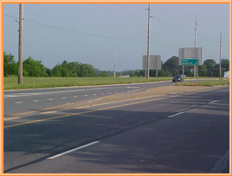
VIEW NORTH FROM ROUTE 10
