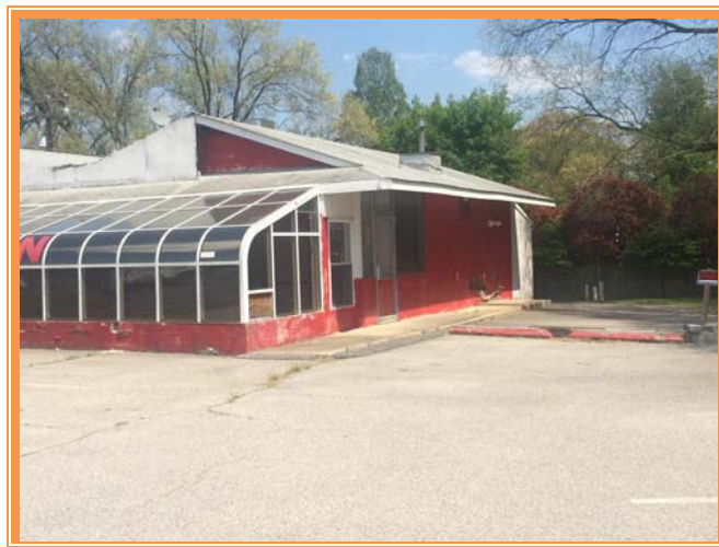
SIDE SOUTH VIEW
